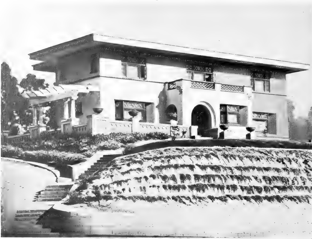
The House of Mr. J. Parkinson, Los Angeles, California
